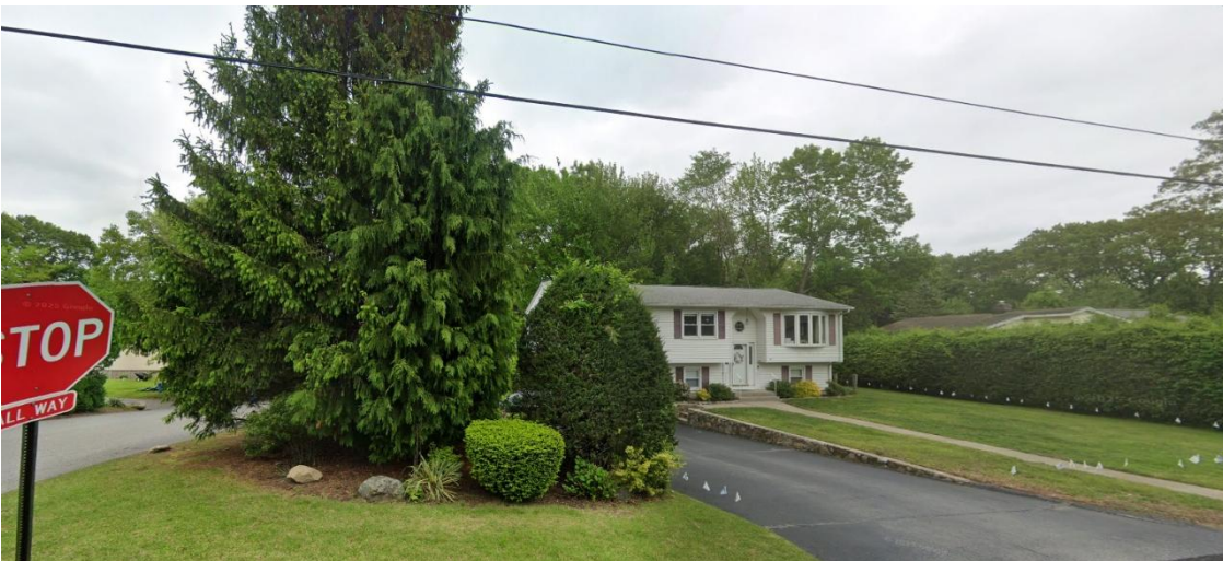
View of Single-family home at 44 Village Ave (Google 2025)
